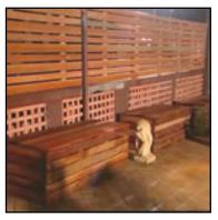
**Balustrade:** Scottie and team Kerba attached a 70x35mm batten to all upright metal posts of the balustrade with 50mm wing tip tech screws. We then horizontally attached Swan River Red (Boral) decking timber, 86x19mm alternating with 64x19mm, to the battens.
